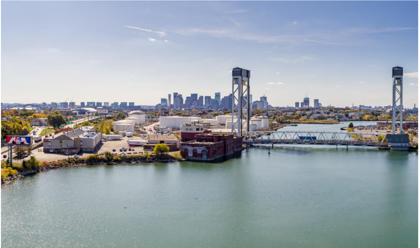
Figure 6: MBTA / MassDOT-owned Railway Site Along Industrial Shoreline of Lower Chelsea Creek 11
