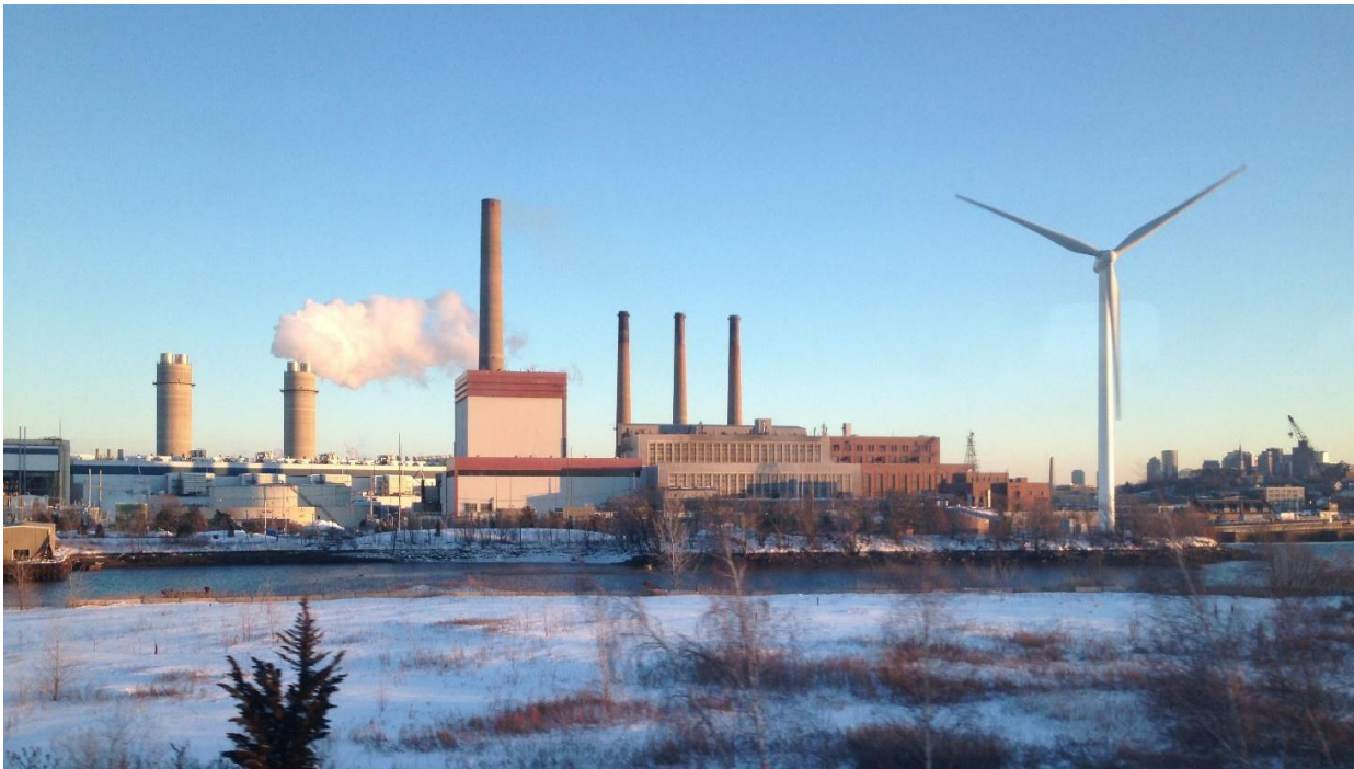
Figure 3: The Mystic Generating Station in Massachusetts 7
